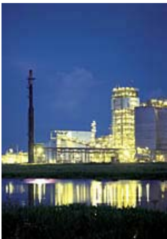
Polk Power Station, IGCC facility, Polk county, FL
