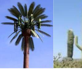
To make cell phone antennas less obtrusive the carriers started to disguise the antennas. The most common disguise is to make a cell phone tower look like a tree. But some places don't have trees such as the Arizona desert or city streets and other disguises are used.
