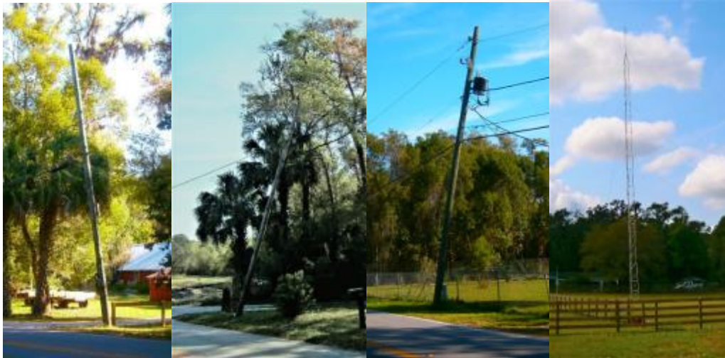
Utility Poles on Grand Ave, Deland
