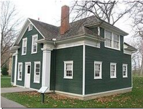
The barn where the gang worked was saved from the wrecking ball and moved to its current location at Moraine Farms, the home of DELCO's co-founder Edward Deeds
