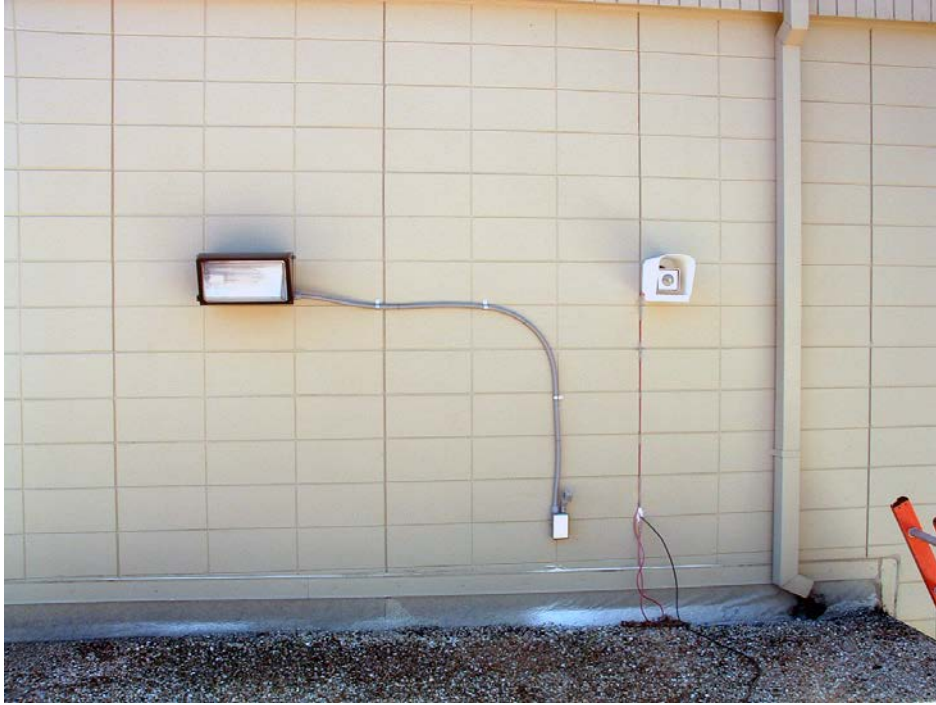
Figure 47 - The completed Halide Flood lamp installation on the exterior wall of the Planetarium
