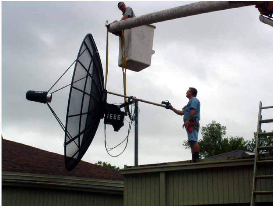
Figure 26 - The SRT is being guided to the mast on the roof of the Daytona Museum of Arts and Sciences
