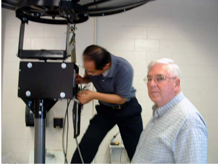
Figure 6 - Dr. Liu installs the remote cabling in the AZ/EL gearbox while Ron Gedney looks on
