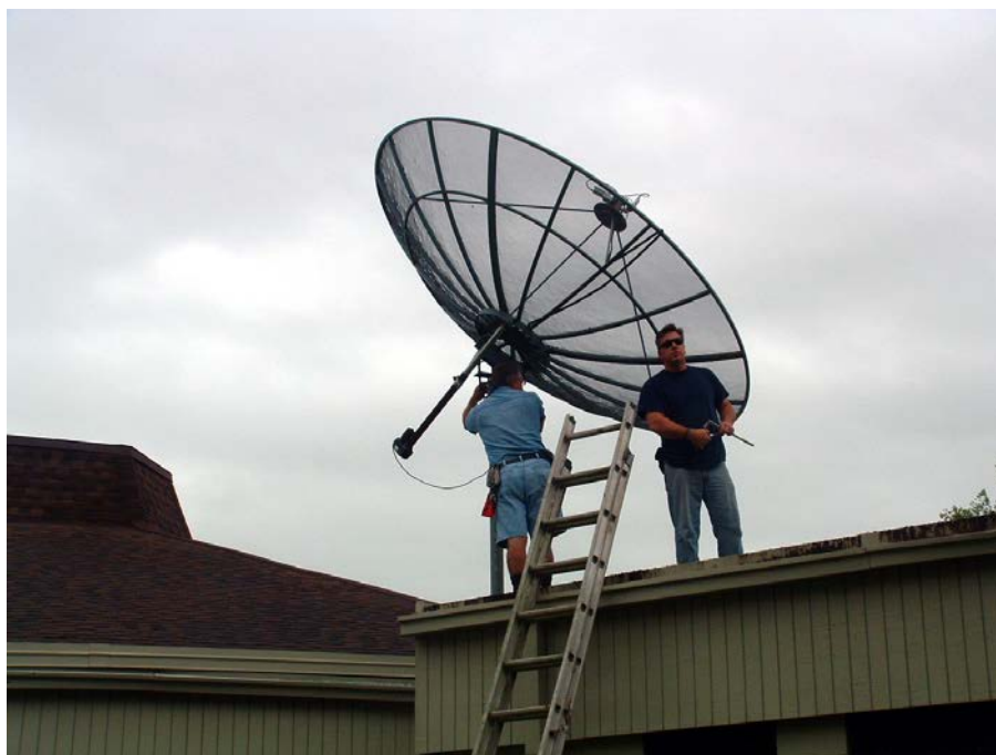
Figure 23 - Removing the "L" Band Satellite Dish from the Antenna Mast
