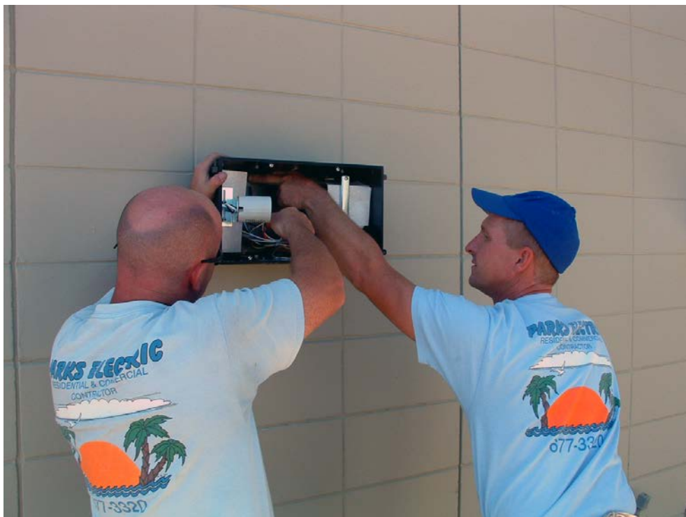
Figure 46 - Mounting the Floodlight fixture on the Exterior Wall of the Planetarium
