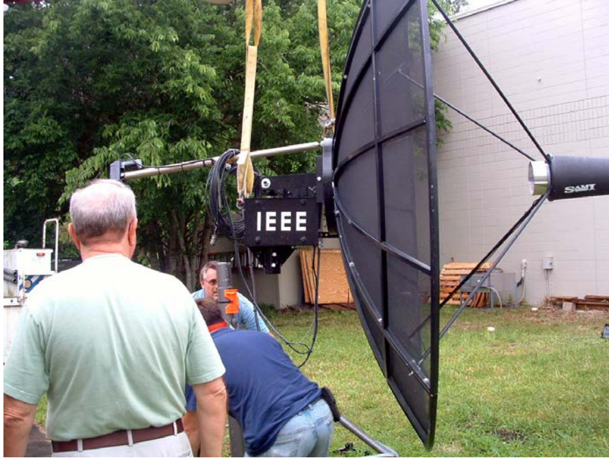
Figure 24 - Lifting the SRT free of the Ground Pedestal
