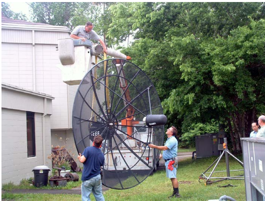
Figure 25 - Moving the SRT from the Pedestal toward the Roof Mast
