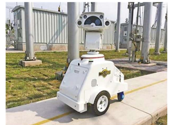
Robotic Substation Yard Inspector 24/7 Outdoor Equipment Maintenance Inspector (Year 2 in service operation)
